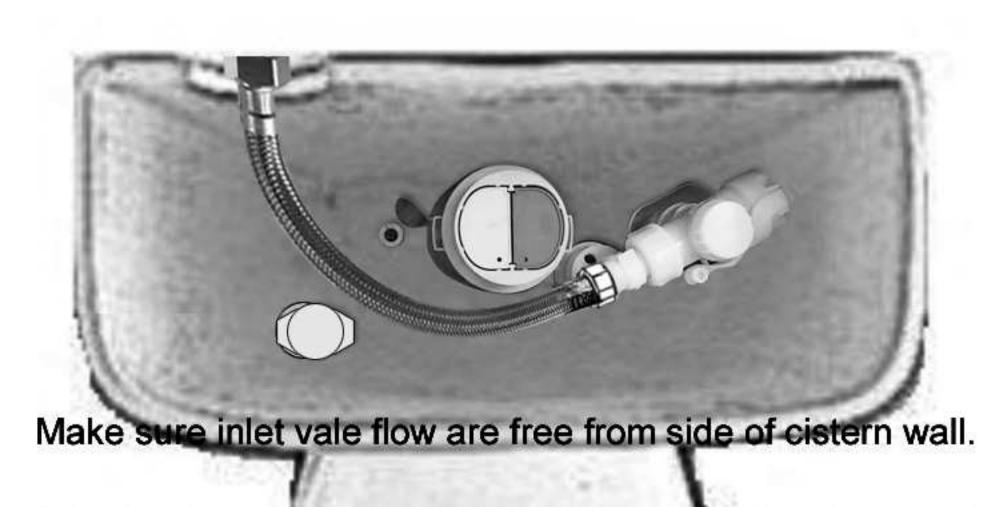
If inlet vale been jam on the cistern wall, it will cause inlet vale keep filling.
